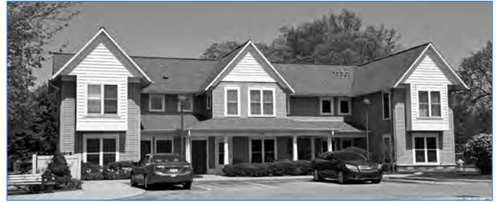
Kingsbury Place Apartments is a 44-unit Dwelling Place development that serves individuals with mental and physical disabilities
