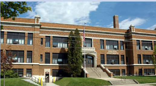
Twenty-unit main building
