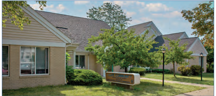
Hope Community Service Center renovations will get underway this fall
