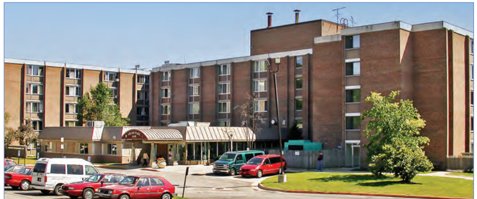
Adams Park Apartments, a 188-unit senior development slated for total redevelopment
