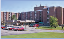
Adams Park Apartments 1440 Fuller Avenue SE, 188 units Low-Income Public Housing Program Ages 62+, people with disabilities
