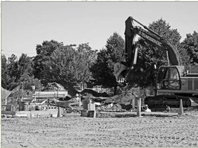
Utility and foundation work begin, August 2020
